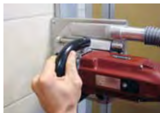
Cut into the tiled wall
