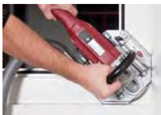
Cut into the corner
