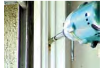
4. Install the new window
