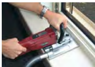
Cut into the window frame
