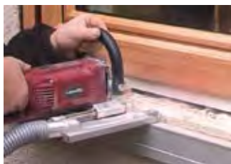
Cut-out for the weatherboard
