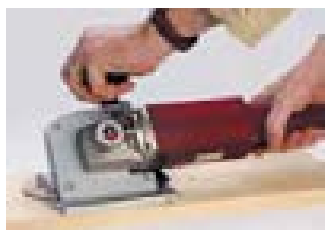
Planing protruding patch
