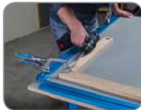
Pocket-Hole Construction
