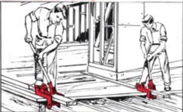
TO TIGHTEN AND TRUE FLOORING
