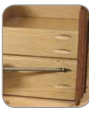
Drive self-tapping screws to secure the joint.
