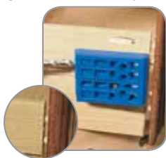
Drill pocket holes at the problem joint.
