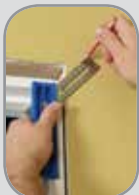
Lay Out Mitered Corners
